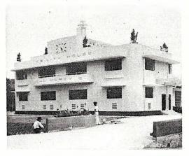
The outer surface of this concrete office building in Singapore. Malaya, is finished with plaster and broken glass particles. Floodlighting makes the building gleam brightly at night.
