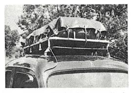
This automobile baggage carrier is instantly removable. It clings to the car top by means of subber vacuum cups that are actuated by suction transmitted from the engine manifold.
