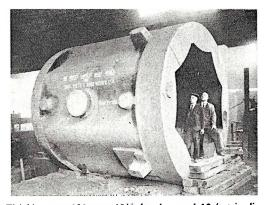
Weighing over 150 tons. 13 $\frac{1}{2}$  feet long and 12 feet in diameter, this ingot mold is said to be the largest in the world. It constituted the biggest single load ever hauled by rail in England and necessitated special rating of freight train.
