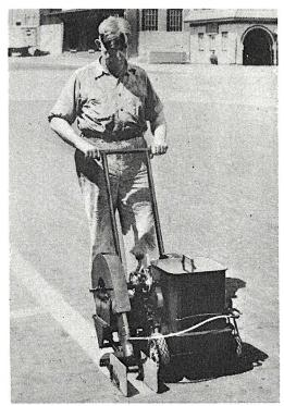
Powered by a % horsepower gasoline engine, this traffic line marker is operated by one man. Paint from the nozzle is sprayed onto the pavement by means of a powerful fan.
