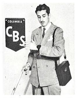
Bob Trout, CBS announces, demonstrates the tiny walking transmitter used for conducting roving interviews. Its parts are concealed in case, wrist strap, money belt, and binocular case.
