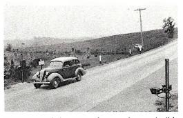
Placed along a highway so passing autos intercept its light beams, this device automatically counts each car and prints a total once every hour. Passing pedestrians do not effect it.
