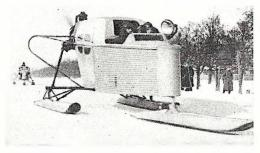
Metal snow-sleds like this one are used to patrol the borders of Soviet Russia. They are powered by airplane engines and propellers and attain speeds not possible with autos.
