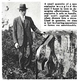
AN EXPLOSIVE that combines safety in manufacture with greater strength and more efficiency in operation has been developed. The powder does not deteriorate with age and no chemical reaction takes place when it is kept in storage.
