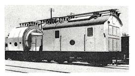
Replacing the old type of stationary power generating stations, these new type mobile generators will provide current for running the fast electric trains of Sweden's main railways.
